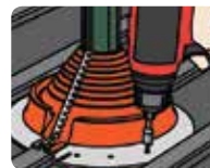
5. Fasten Retrofit to roof.
