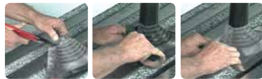
1. Trim to Fit 2. Wrap and Snap 3. Press and Mold
