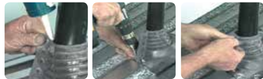
4. Add Urethane Sealant. 5. Fasten 6. Install Cable Tie Sealant.
