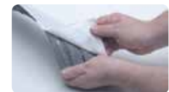
Pre-applied adhesive helps to keep closure in place before roof panel is fastened.
